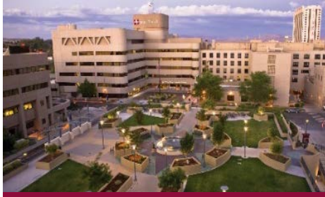
Saint Mary's Regional Medical Center, Reno, Nevada
